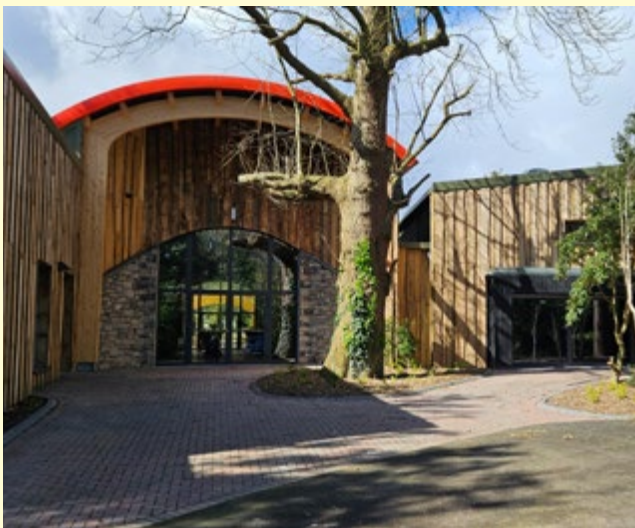
(Above) Entrance to the new Education, Conservation and Research Centre at Fota Wildlife Park (Above right) Lecture theatre inside the Education, Conservation and Research Centre
